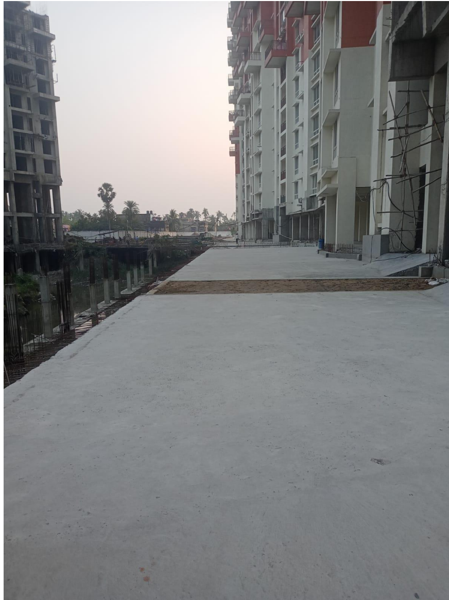
Deck Slab behind Block 8-9-10
