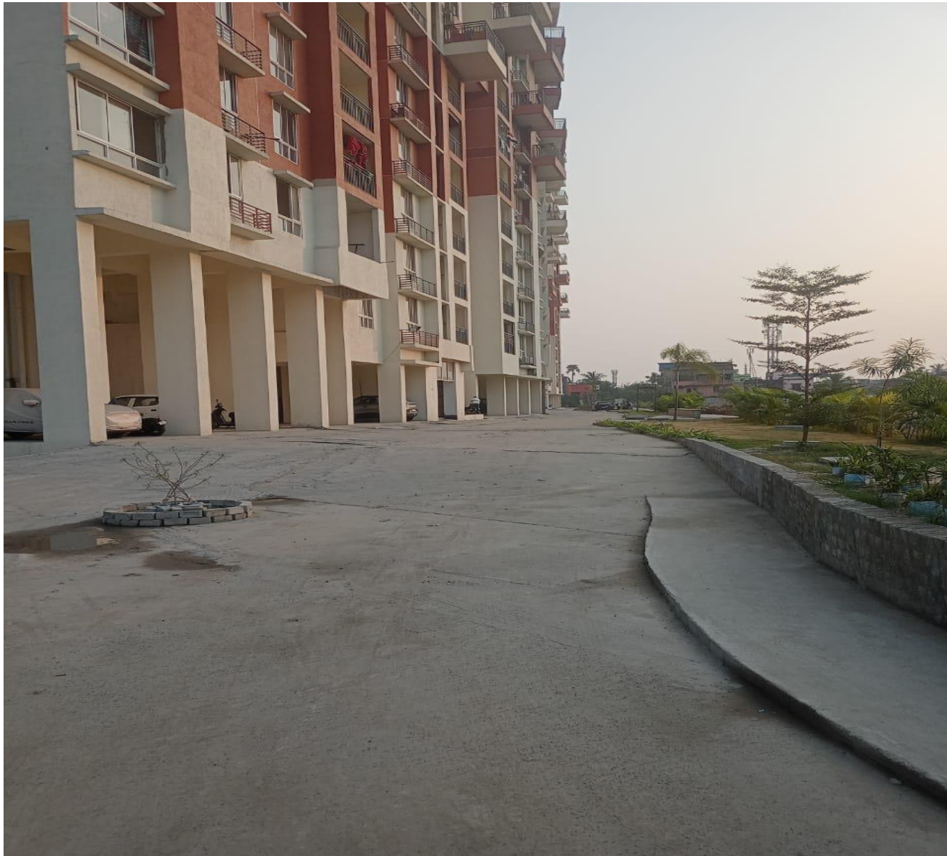
Driveway in front of Block 8-9-10
